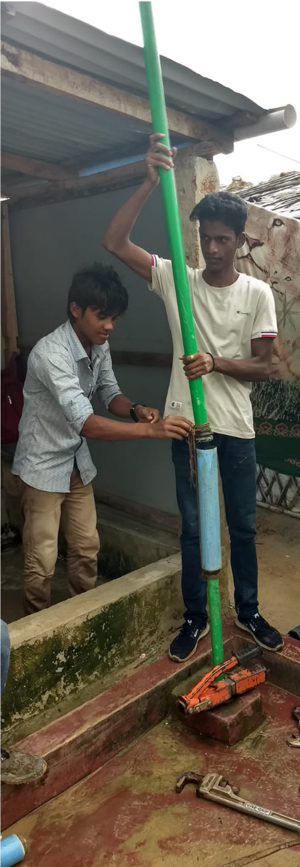
Picture of Anise and Shahed repairing a well in the rain. This shows how their rope tying technique successfully prevented the cylinder from falling down into the well. Even though the threads stripped out from the PVC cylinder, the rope kept it tied on to the pipe.
